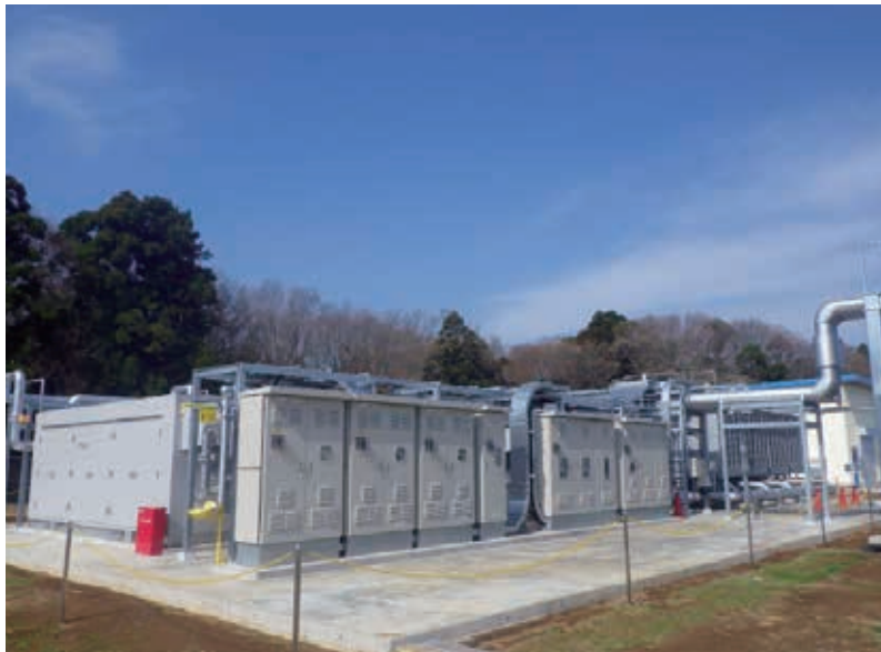
Ammonia refrigeration system for the KIT KAT line installed at the Kasumigaura Factory in 2015
